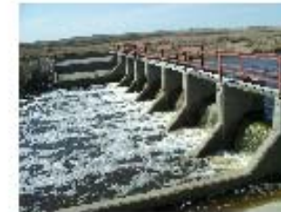
The Elie Dam, one of 8 major water control structures in the La Salle River Watershed.
