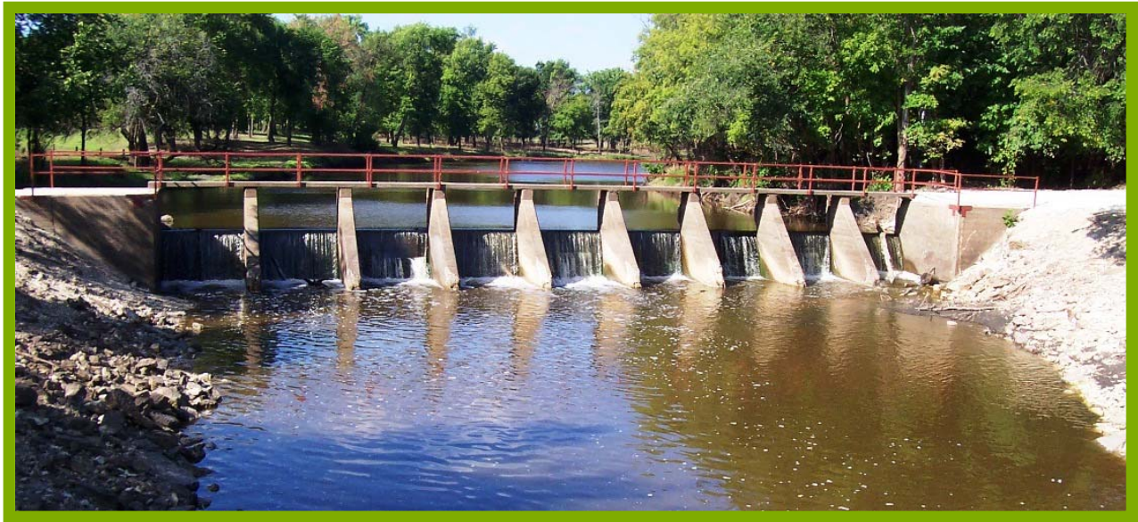
St. Norbert Dam
