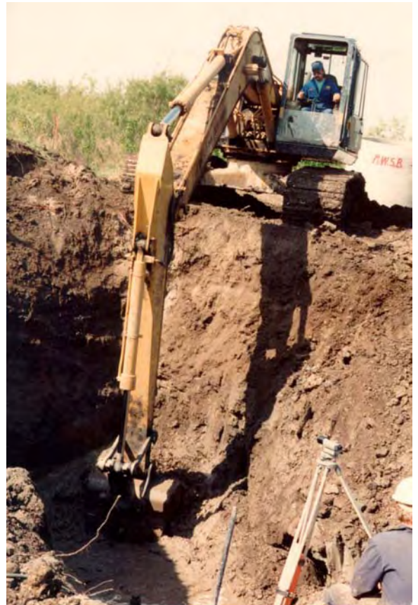
Backhoe installs wet well
