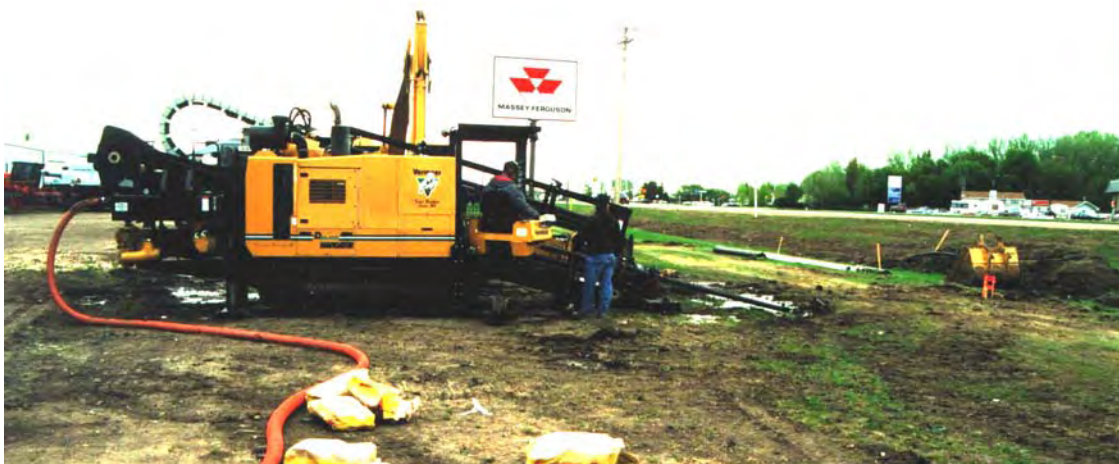
Pipeline is tunnelled under highway.
