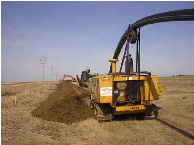
Trencher installs pipeline.
